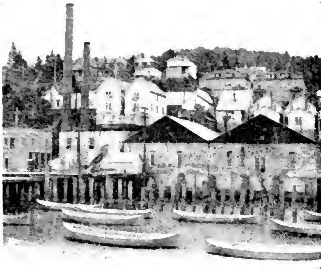
Astor Street Generating Station at Astoria - July, 1910
